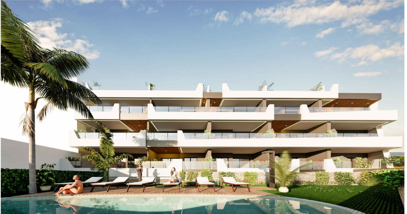
03178 Benijofar | Costa Blanca South | Project | Referentie: CBLS11870-15007
